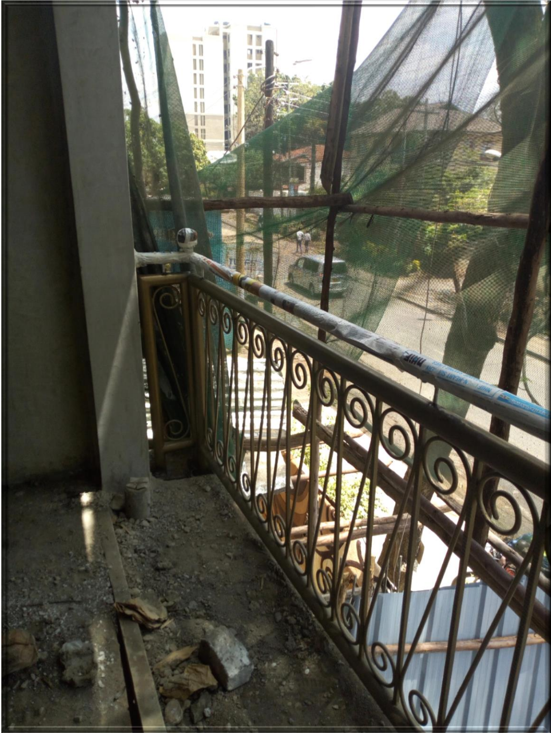
Fig. O5. Fabrication properly protected in progress as below
