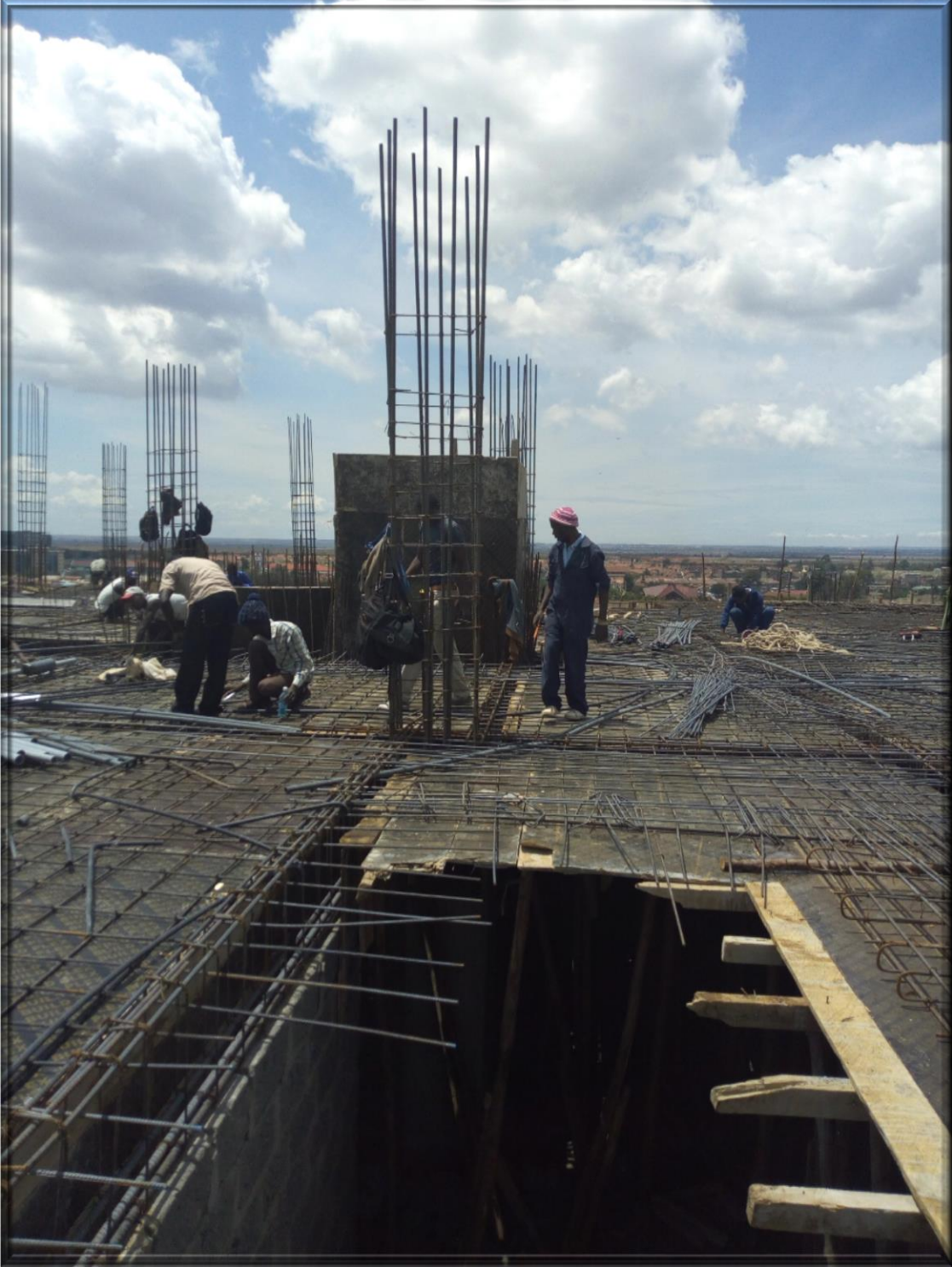
Fig. 03. Lift shaft preparation for formwork and steel fixing in progress
