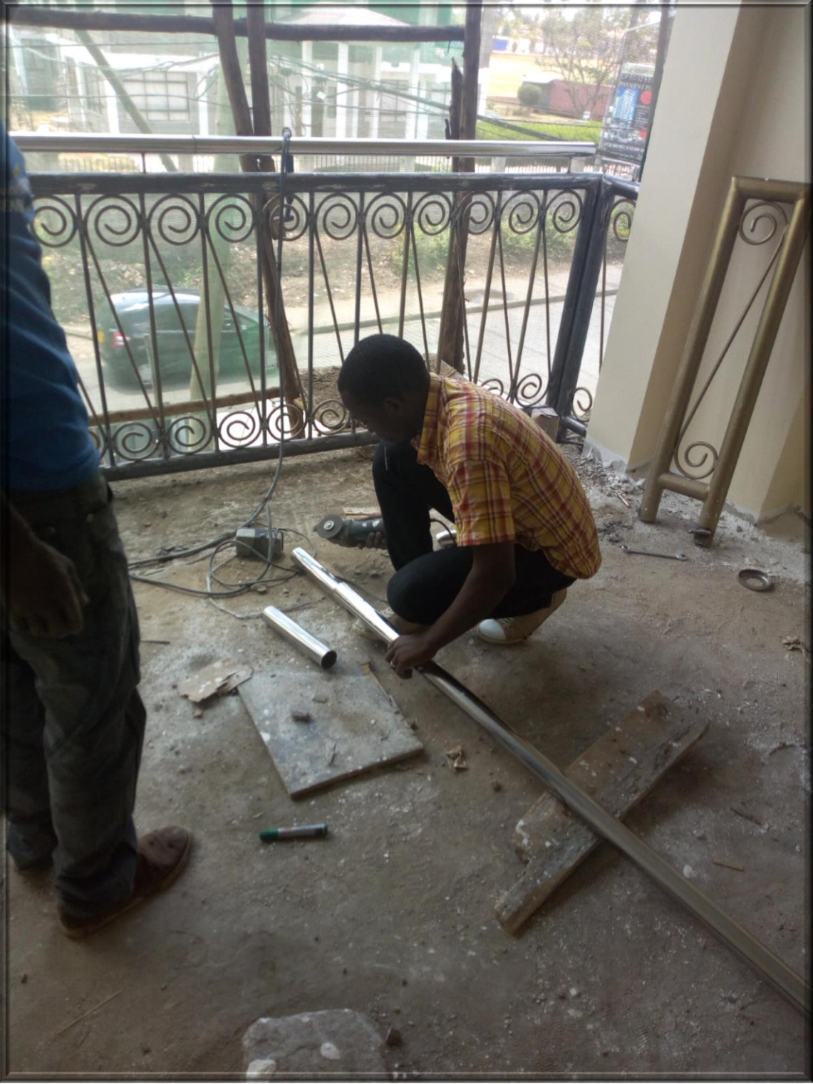
Fig. 04. Welding and fabrications for first floor sample works on going
