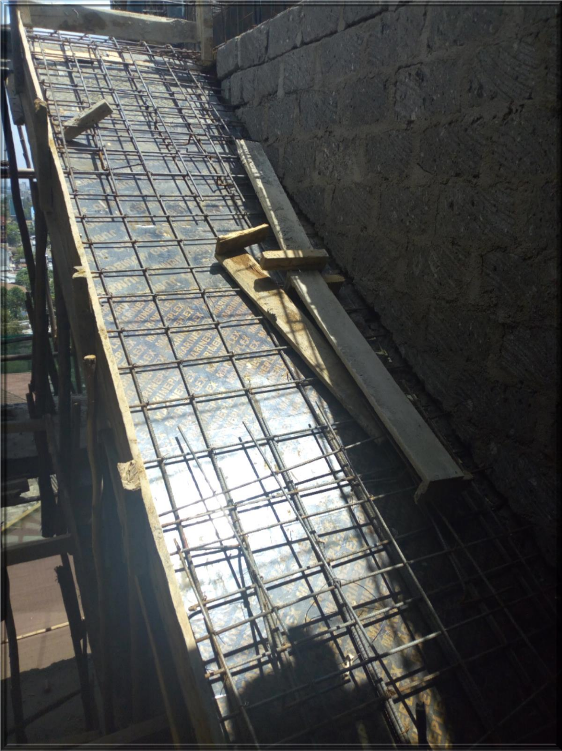
Fig. 02. 10 th Floor stair steel and formwork in progress
